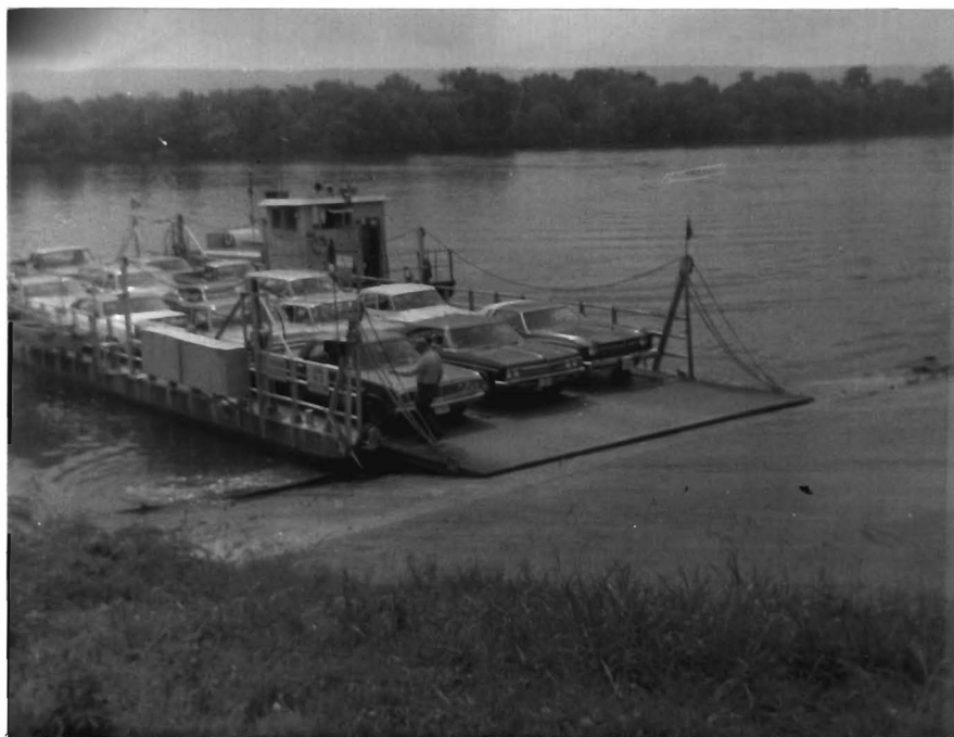
Figure 14. The South Pittsburg Ferry completing a crossing on the Tennessee River.
